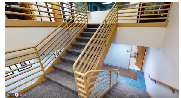
Rear Egress Stair
