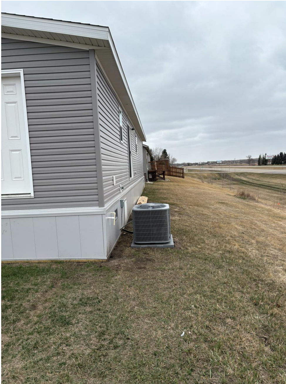
Back view of place home – in line with neighboring houses
