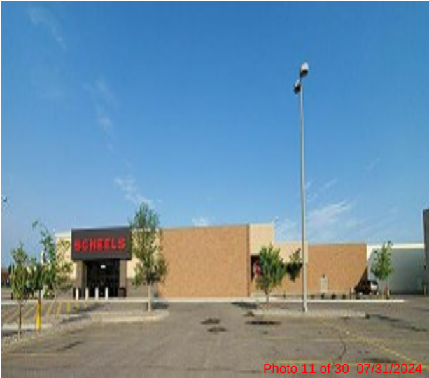
Property attached to subject property on southwest corner platted on dif
