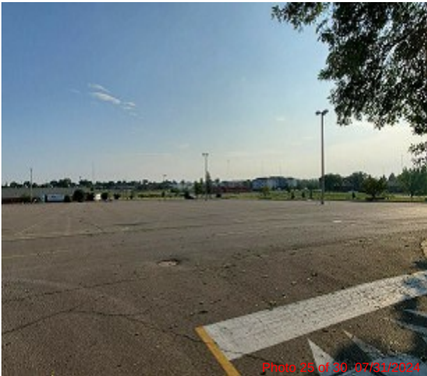
Parking lot scene looking northeast from east side of the building.
