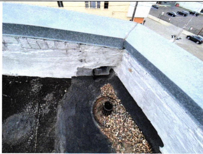
A-3 #1 Mastic, fabric and coat scupper
