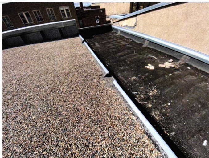
A-3 #2 Clean & coat scuppers
