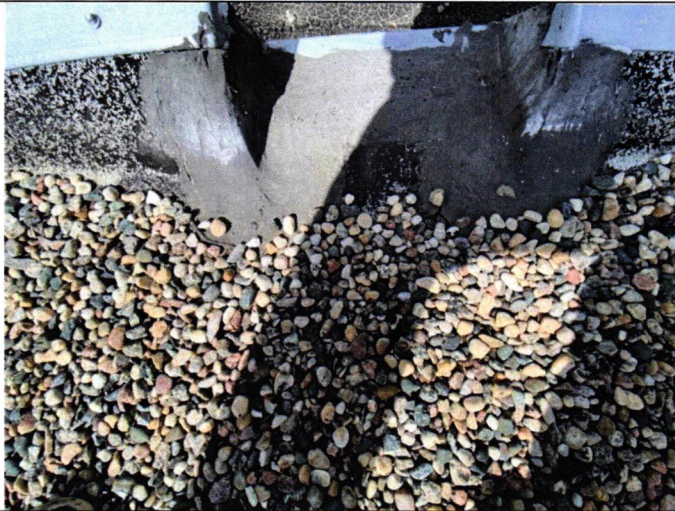
A-3 #2 Clean & coat scuppers
