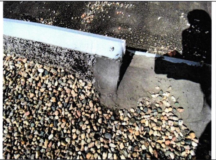
A-3 #2 Clean & coat scuppers
