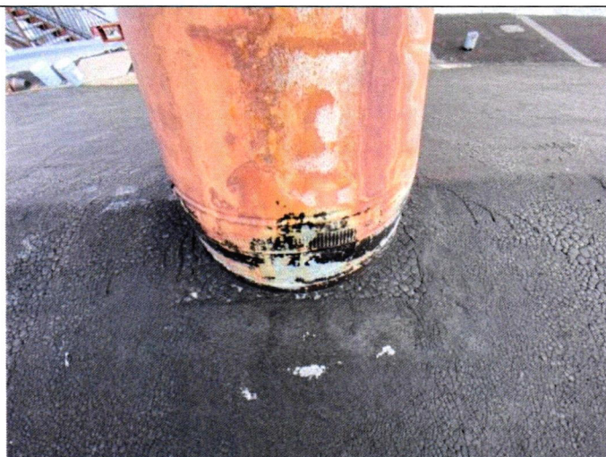
A-3#4 Clean and coat bottoms of stacks
