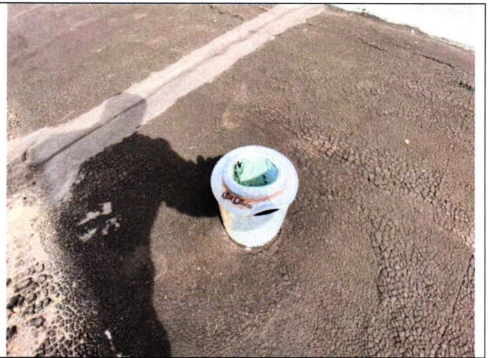
A-3 #5 Repair open lead top
