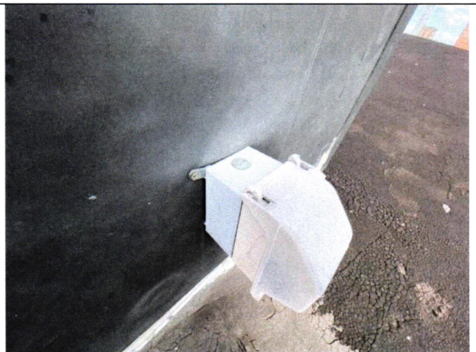
A-3 #3 Seal screws on wall flashing
