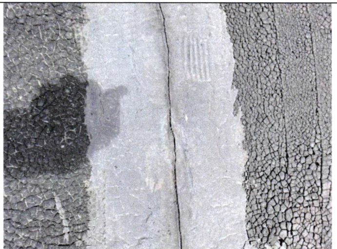
A-3 #2 Coat and seal seams
