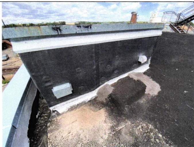
A-3 #3 Seal screws on wall flashing
