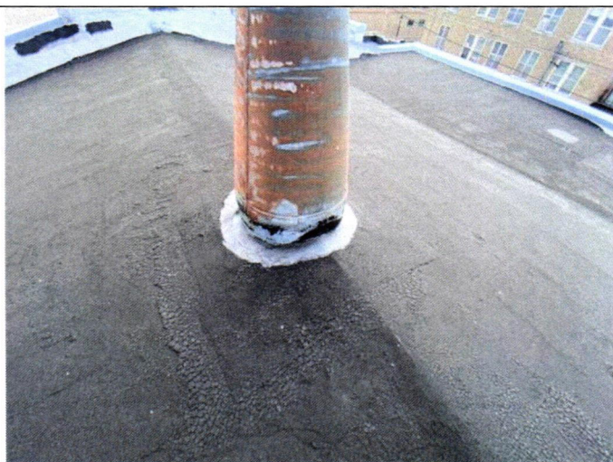
A-3#4 Clean and coat bottoms of stacks
