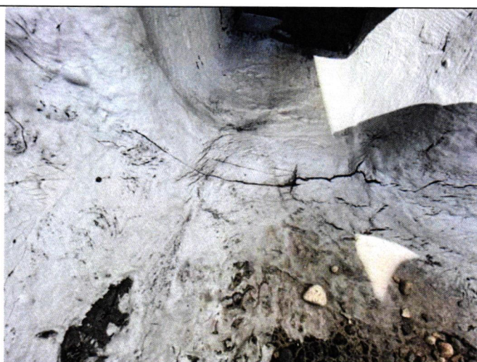
A-3 #1 Mastic, fabric and coat scupper
