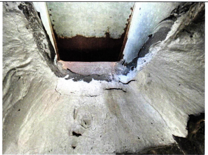
A-3 #1 Mastic, fabric and coat scupper
