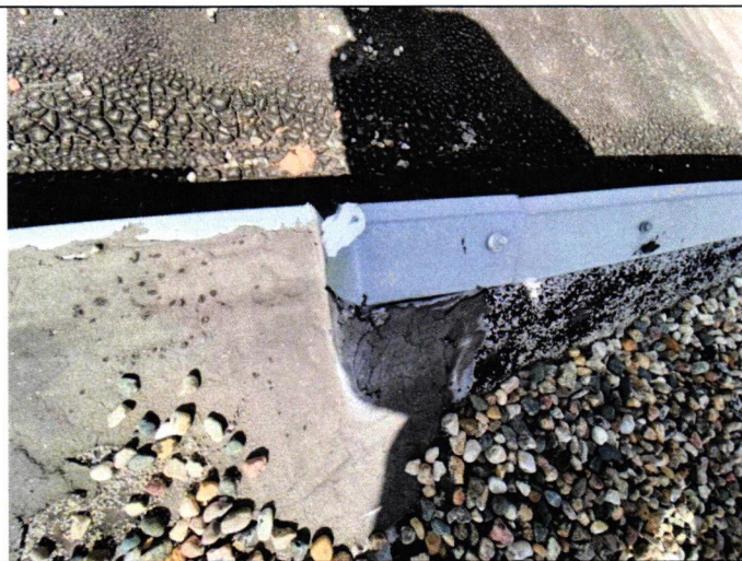
A-3 #2 Clean & coat scuppers
