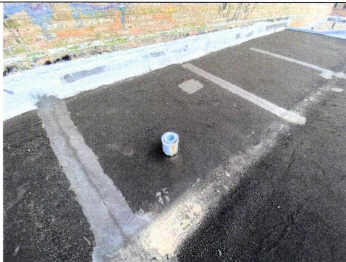
A-3 #2 Coat and seal seams
