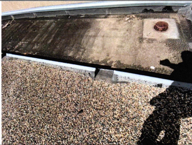
A-3 #2 Clean & coat scuppers
