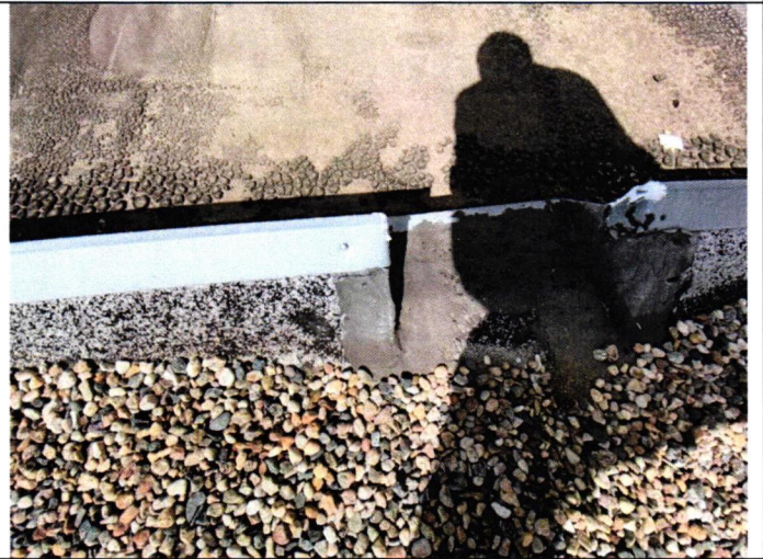
A-3 #2 Clean & coat scuppers
