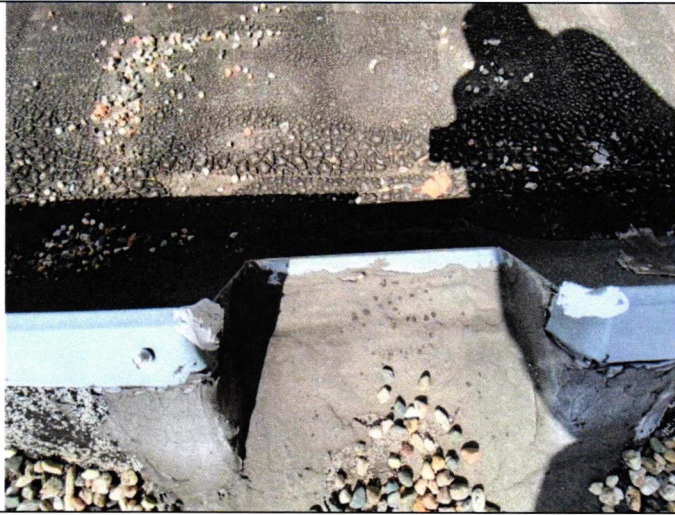
A-3 #2 Clean & coat scuppers
