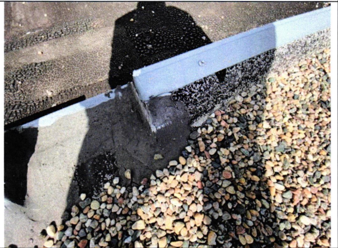
A-3 #2 Clean & coat scuppers
