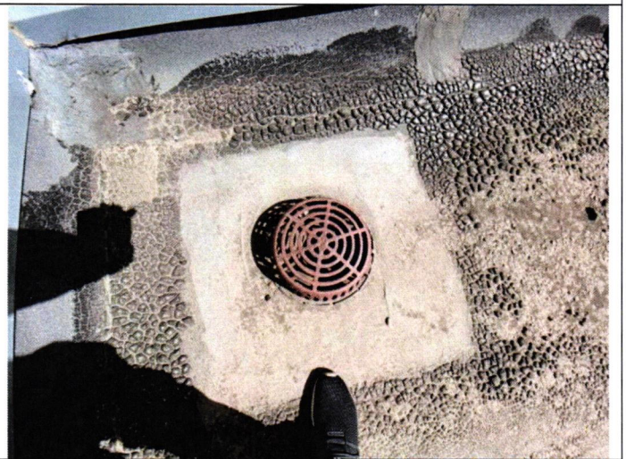
A-2 #1 Clean and re-coat drain area
