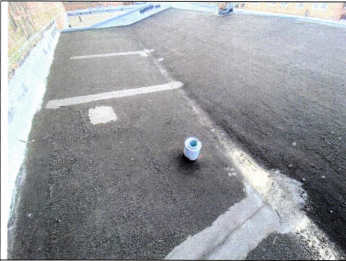
A-3 #5 Repair open lead top
