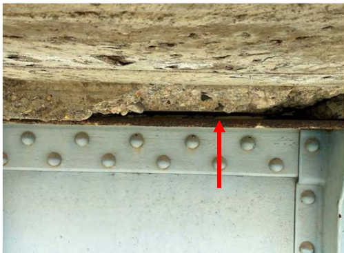
Deck Separation at Pier 9
