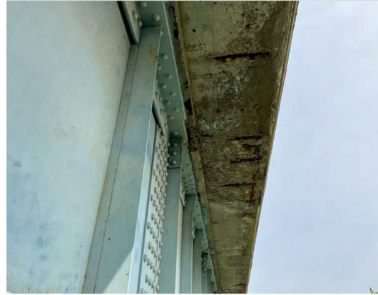
Bridge Deck Overhang
