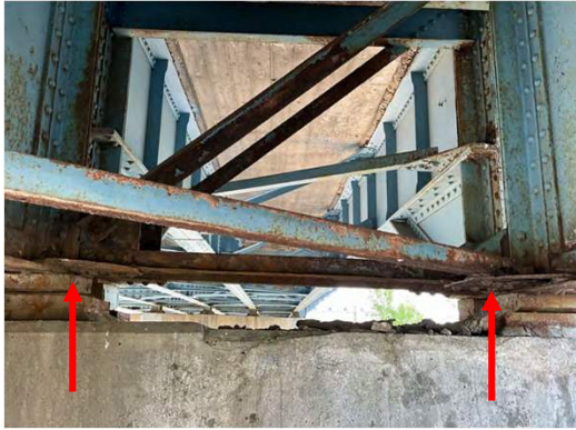
Gusset Plate Section Loss
