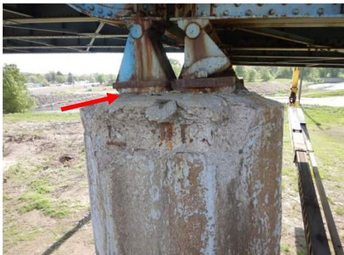
Bearing Undermining
