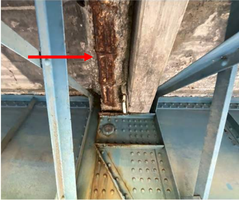
Span 9 Drop Slab
