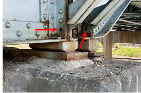
Missing Rivets from Pack Rust
