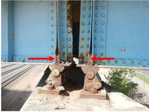
Pack Rust at Bearing Stiffener
