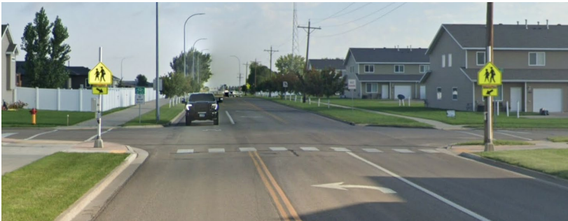
Figure 8 - RRFB System on 13th St SE near Hoeven Elementary
