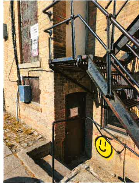
Rear Basement Door
