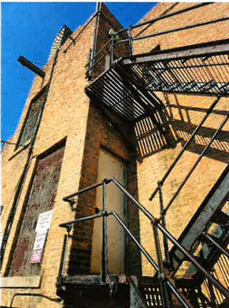
Rear Fire Escape
