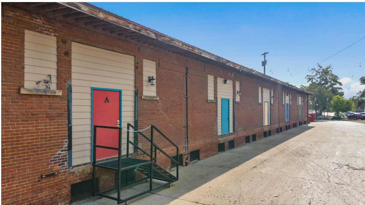
EXISTING BUILDING CONDITIONS
