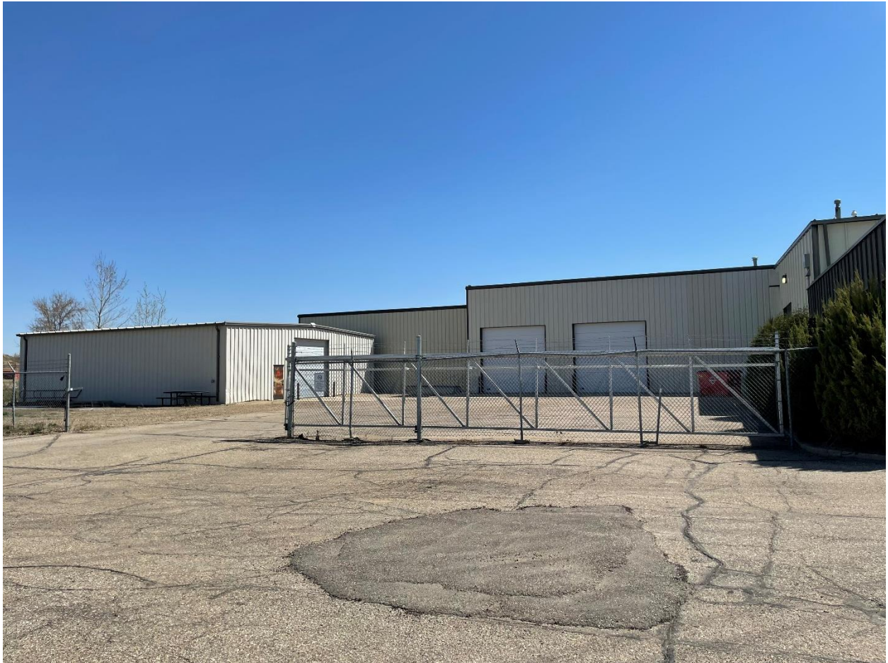
Facing East – Building to house hazardous materials (3100 4 th Ave SE)
