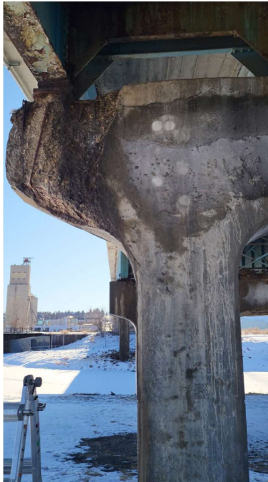
Pier 3 North Face East Column
