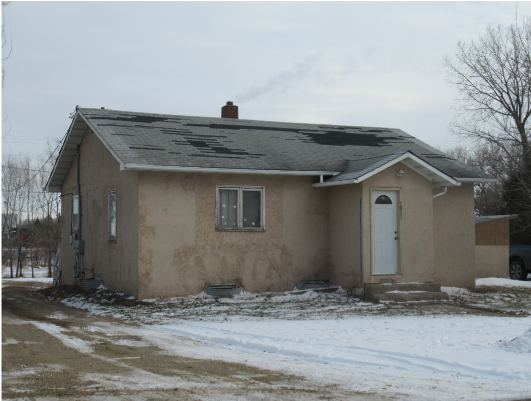
1 Story to the North:
