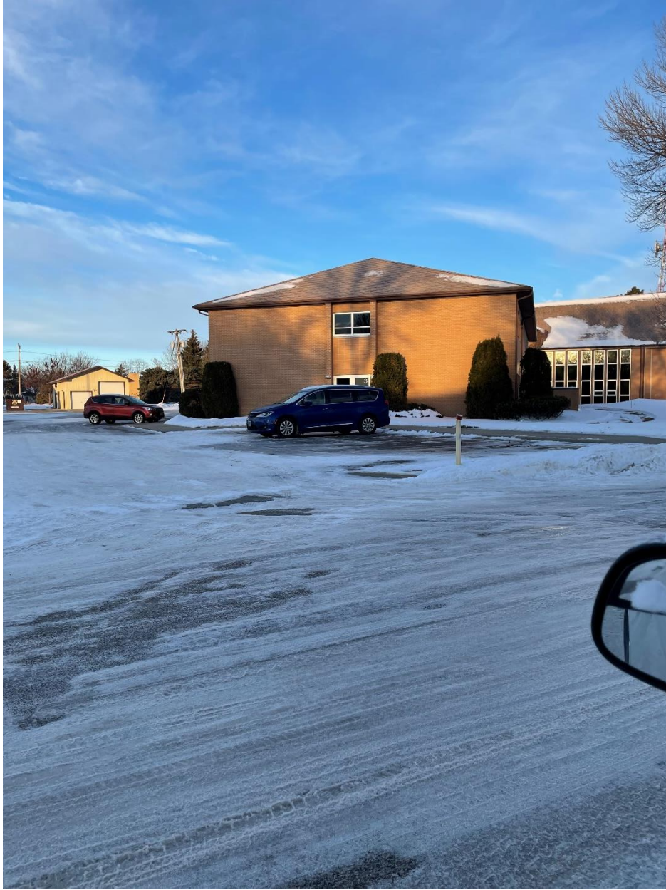
Facing Northwest – Building addition area
