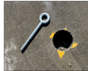
Eye-Bolt Pictured with nut removed.
