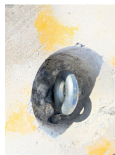
Eye-Bolt in Seated position after completing steps 2, a. and 2, b.
